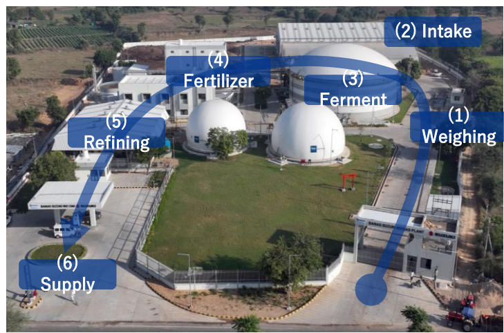
Bhukhala Biogas Plant
