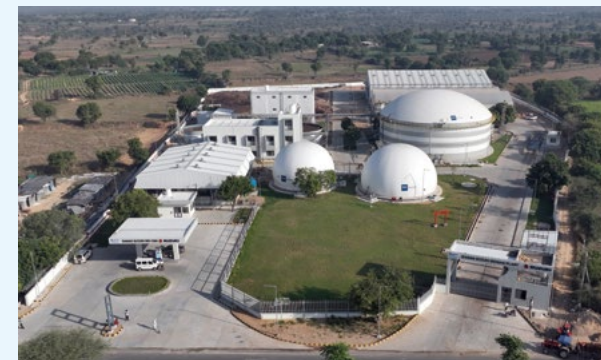
BANAS SUZUKI BIOGAS PLANT
