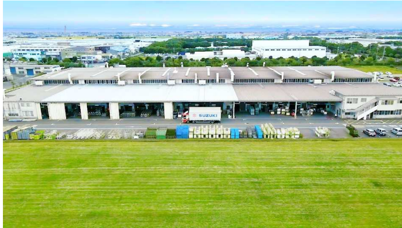
Plant owned by the Suzuki Group in Iwata, Shizuoka
