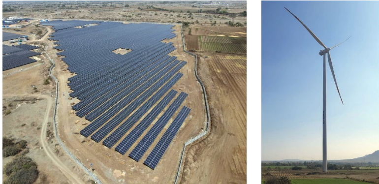
Power generation facility for SMG (Provided by ReNew Power Private Limited)
