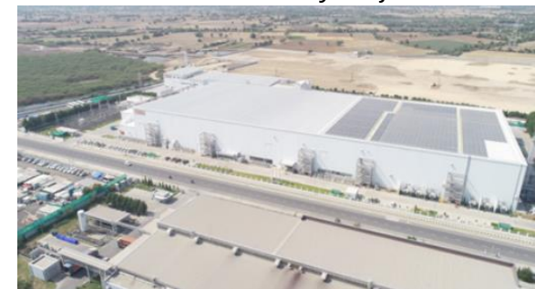
TDS Lithium-Ion Battery Gujarat Pvt. Ltd.
