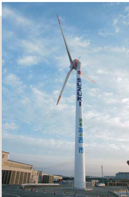
Wind turbine generator in Kosai Plant
