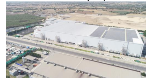
TDS Lithium-Ion Battery Gujarat Pvt. Ltd.
