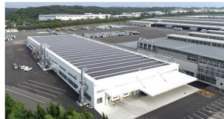
(5) New inspection building
