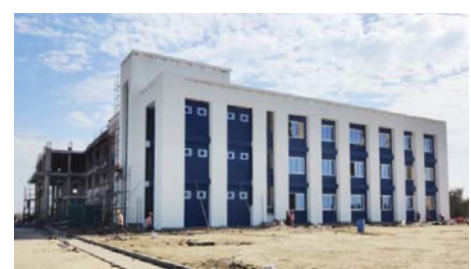
School in Sitapur, Gujarat under construction
