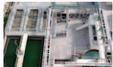
A wastewater treatment facility newly installed and operated in June 2007
