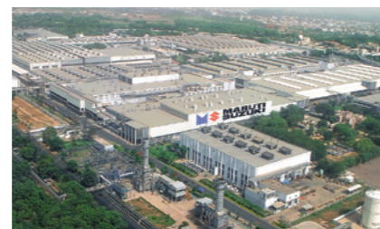
32 MARUTI SUZUKI INDIA LIMITED (India) GURGAON PLANT
