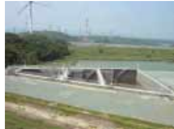
Kosai Plant: Emergency Retention Tank (Capacity: 4,800 cubic meters)
