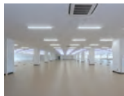
Installation of LED lights
