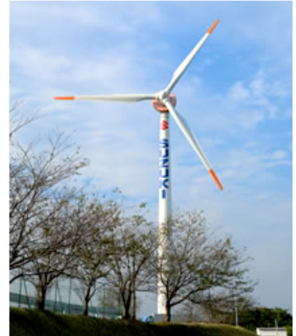
Wind power facility at Kosai Plant
