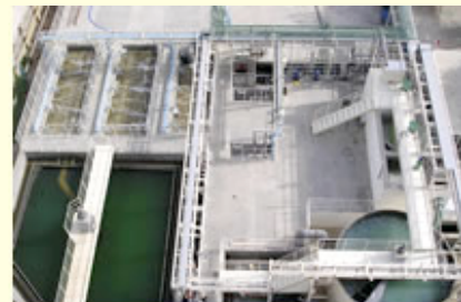
A wastewater treatment facility newly installed and operated in June 2007
